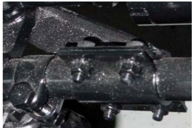
Close-up of support brace
